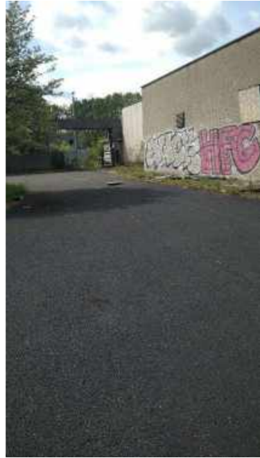
The Existing Building on the Eastern Side of the Site
